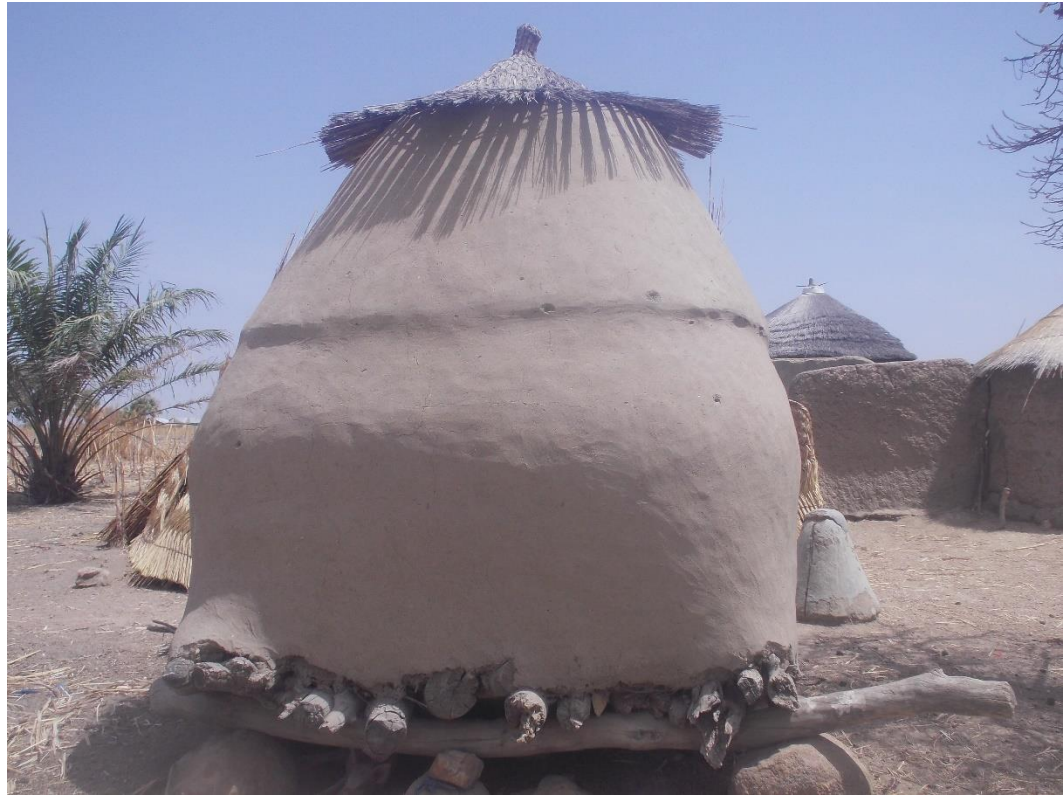
Figure 46: Barn/silo (Baare/Boore) for the storage of food, particularly cereals at Apotdabogo II.
