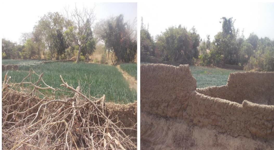
Figure 47: Mud fence built around farms at Gabuliga
