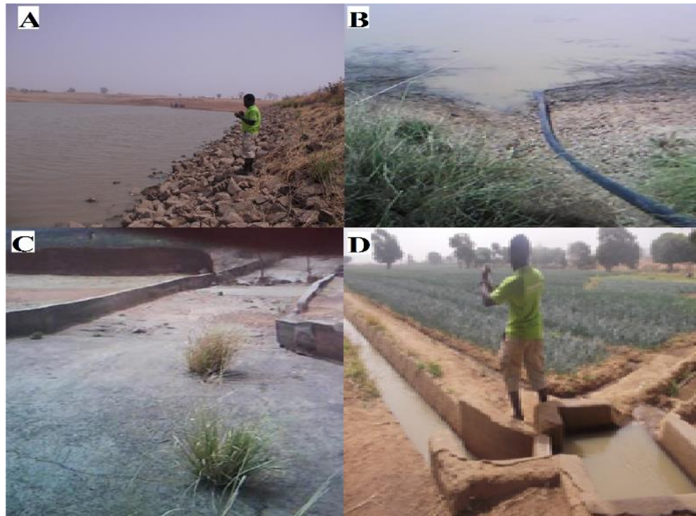
Figure 34 (A&B): Tube and canals to source water from dam to farms at Kuka; (C) – Irrigation channels at an onion farm at Kuka.
