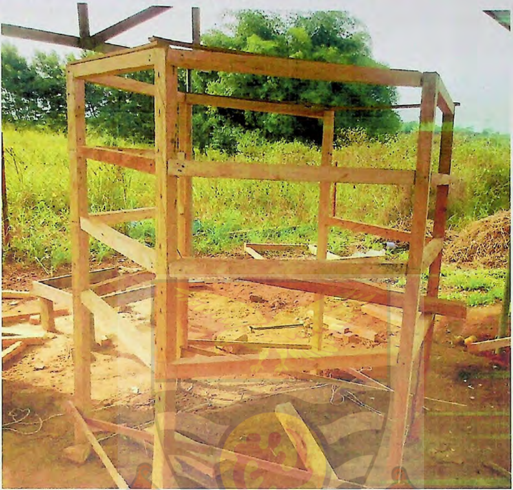
Figure 28: Construction of hexagonal evaporative structure (HexB)
