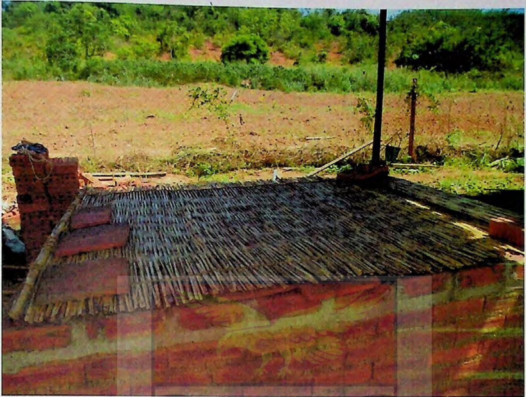
Figure 19: Brick-walled Cool Chamber (Evaporative structure) with thatch cover
