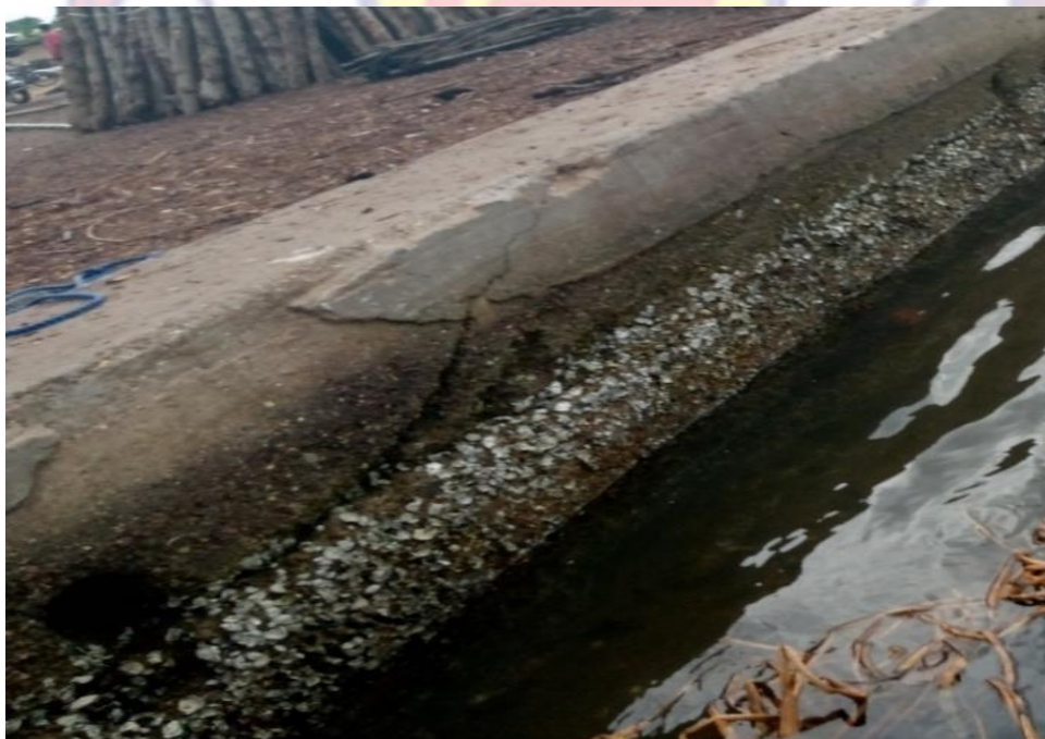
Figure. 3.4: Spat of oysters settling on the concrete wall built at the landing site on the Volta estuary (Anyanui).
