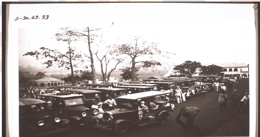
Figure 3. 3 Lorry Park Kumasi
