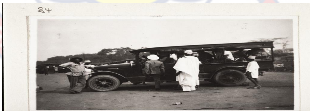
Figure 3. 1 Lorry Park, Kumasi 1925
