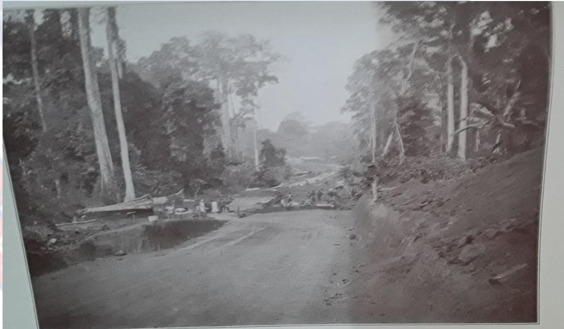
Figure 2. 6 Tarmet – Construction work on Road A7. Asante 1923
