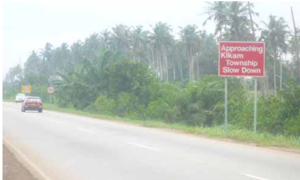
Plate 3: Ankobra- Kikam stretch of road with sign post
