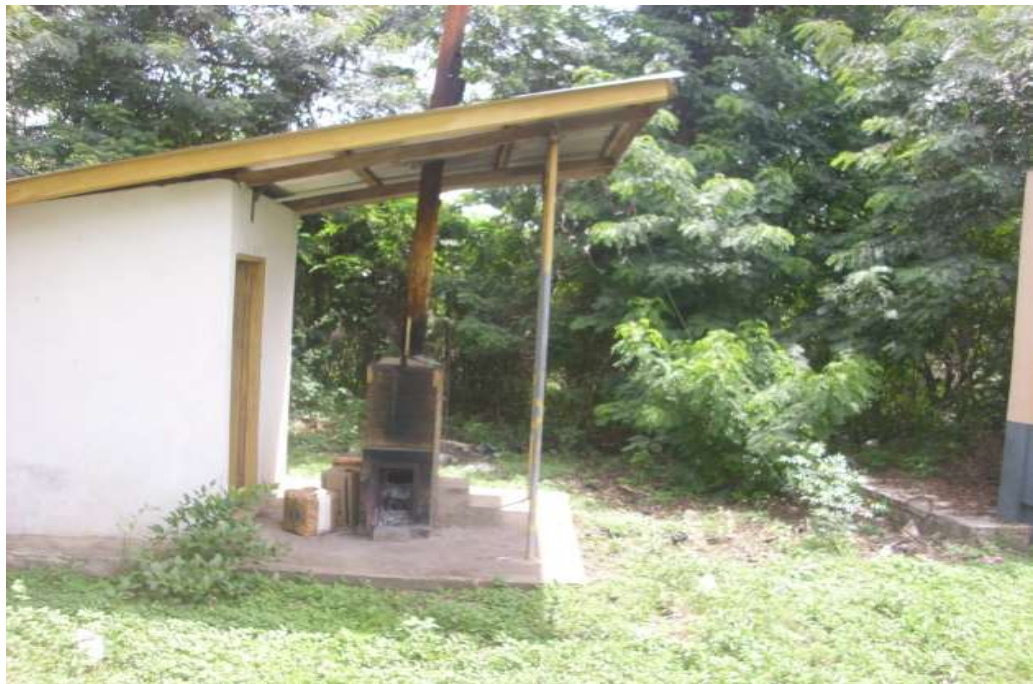
Figure 16: A De-Montfort incinerator used by Donkorkrom hospital
