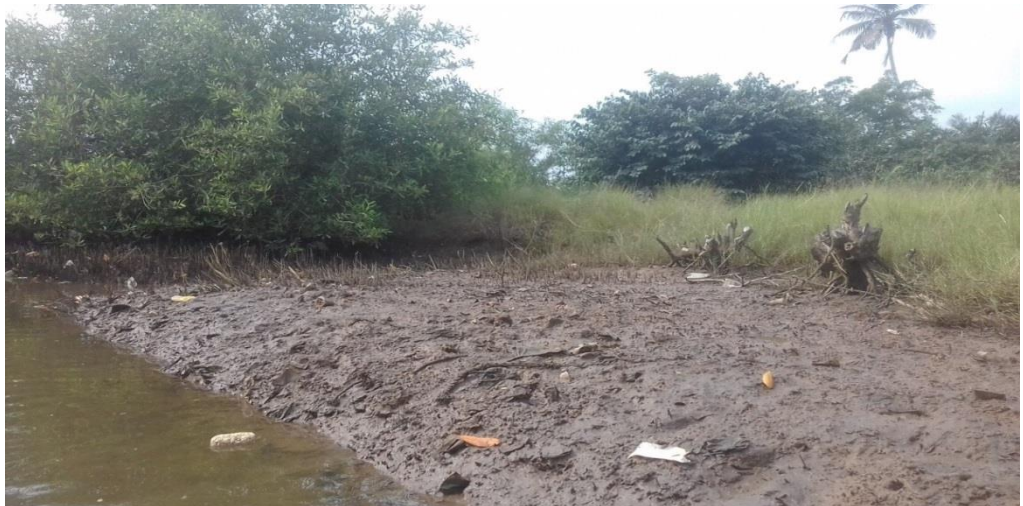
Plate 30: Degradation and forced deposition along the banks (lower section)
