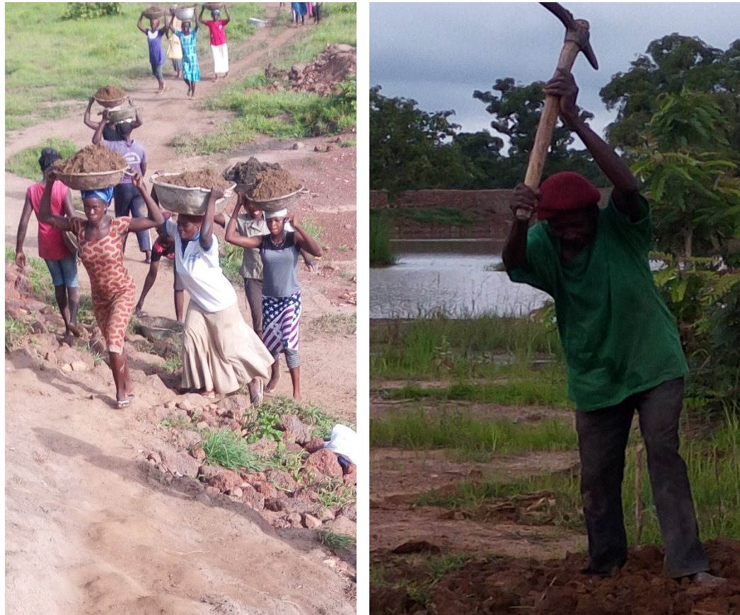
Figure 17: Women transporting sand and a man digging sand at the Poyentanga dugout rehabilitation project Source: Field survey(2017)
