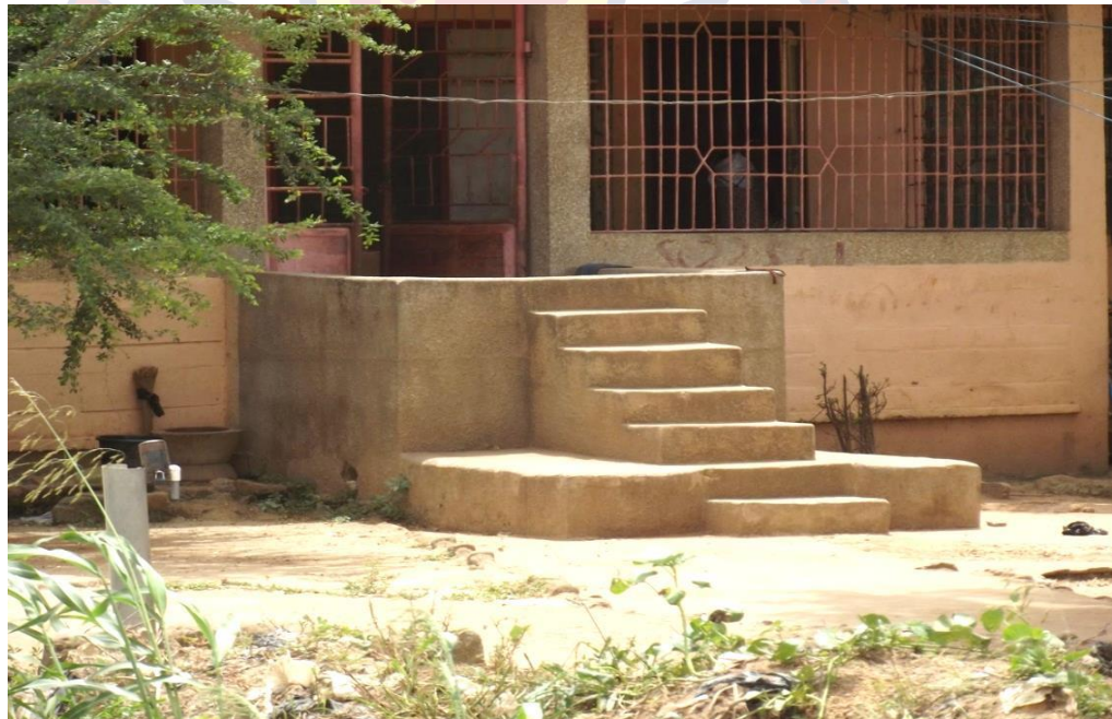
Plate 4. 13: A flight of stairs constructed to protect a house from floods, Accra. Source: Author 2014, Field Survey.
