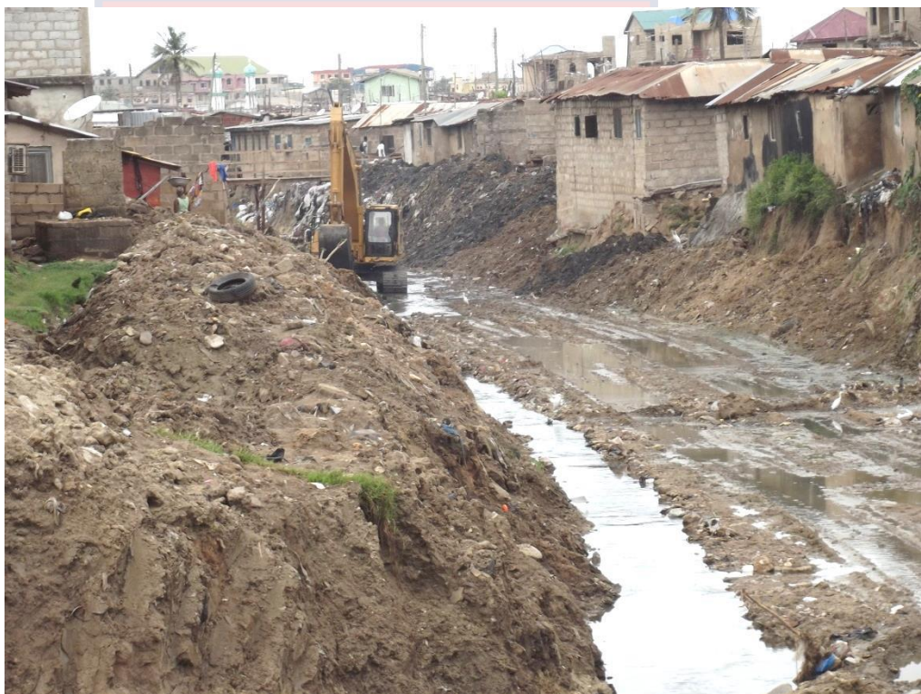
Plate 4. 9: Dredged and widened Stormdrain in a suburb of Accra. Source: Author 2014, Field Survey
