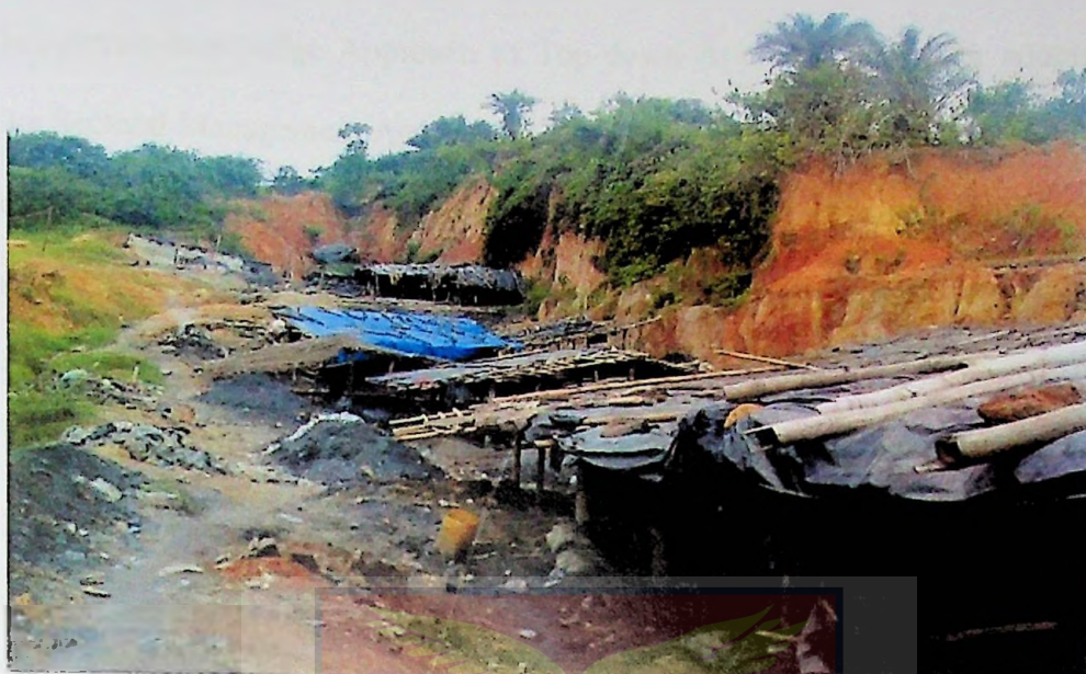
Figure 14: Fragile structures built to control erosion in the basin Field data (2016)
