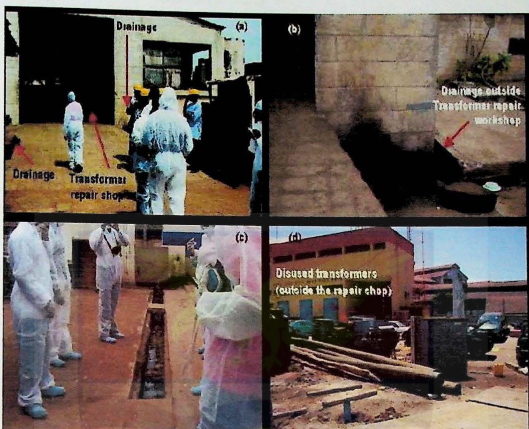
Plate 8: Potential contaminated sites identified at ECG transformer servicing center in Accra (Centeno, 2010)
