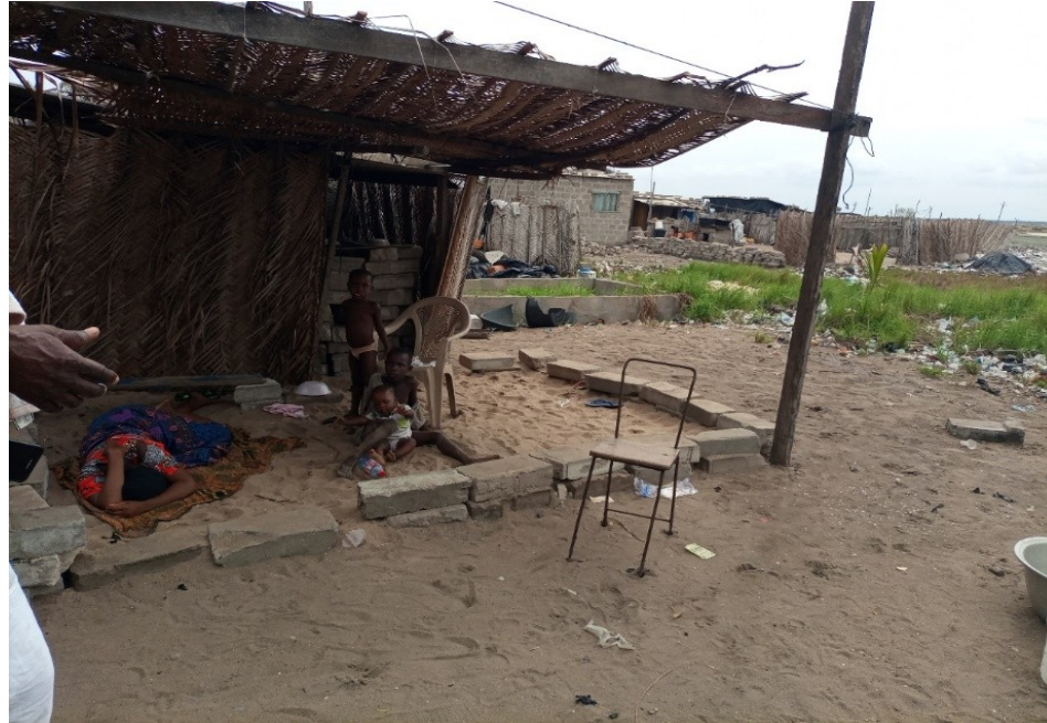
Figure 26: Houses that have been relocated into the dry areas of the Keta Lagoon.
