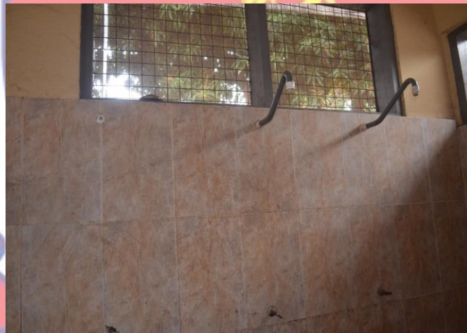
Figure 20: UG Changing Room with shower
