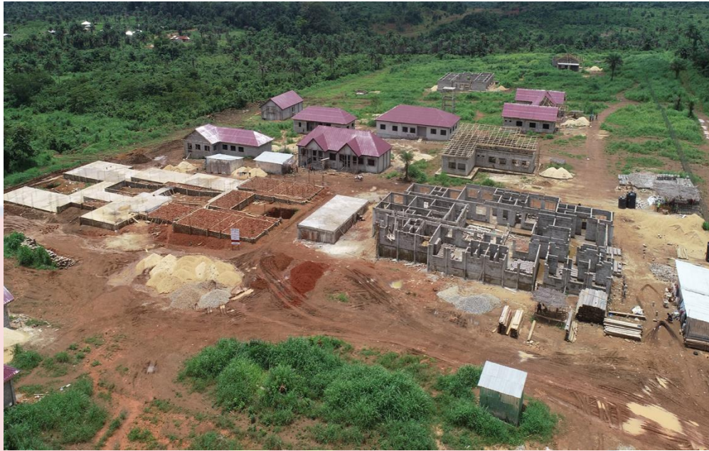
Plate 7: 100-Bed Community Hospital Under Construction, Ngolala
