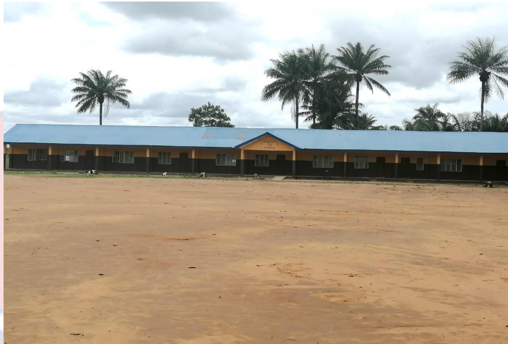
Plate 9: Newly Constructed School at Kangahun, Lower Banta Chiefdom Photo credit: Author (2022)
