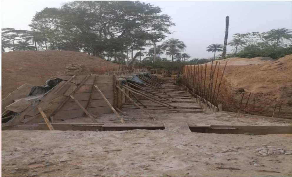
Plate 2: Road Diversion Due to Culvert Construction, Taninihum
