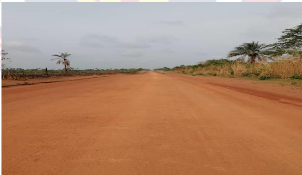
Plate 3: Constructed Feeder Road in Gondama
