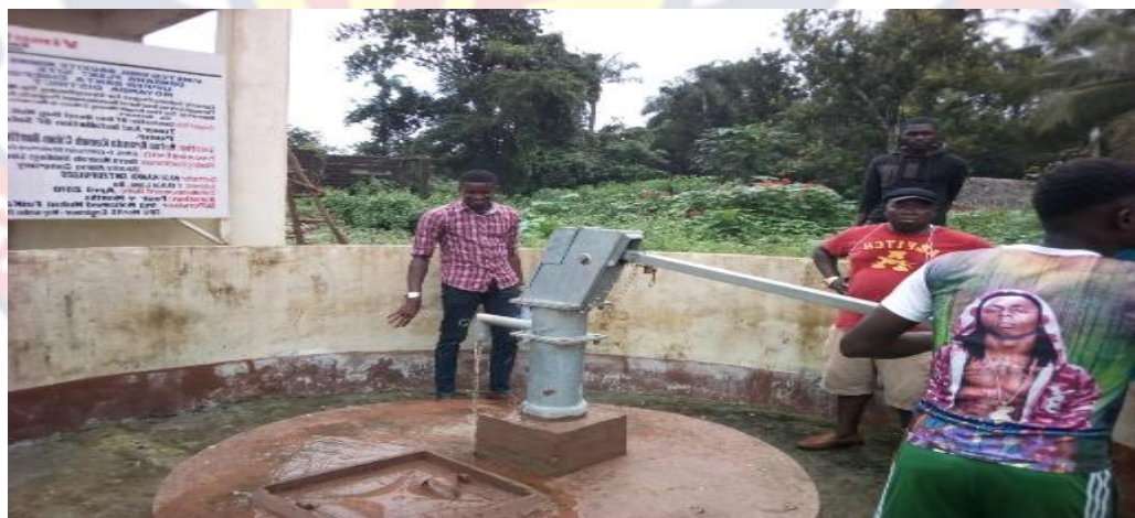
Plate 14: Bore Hole at Ngolala, Upper Banta Chiefdom
