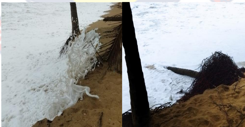
Figure 55: Coastal erosion leading to eroding of coconut trees at Ibeju-Lekki
