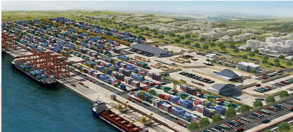
Figure 7: An Artist's Impression of Lekki Deep Sea Port ( https://areteafrica.com/2022/03/11/lekki-seaport-construction-nears-completion )
