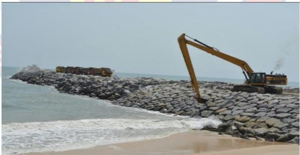
Figure 51: Stone pilling construction for cargo landing at the Ibeju-Lekki
