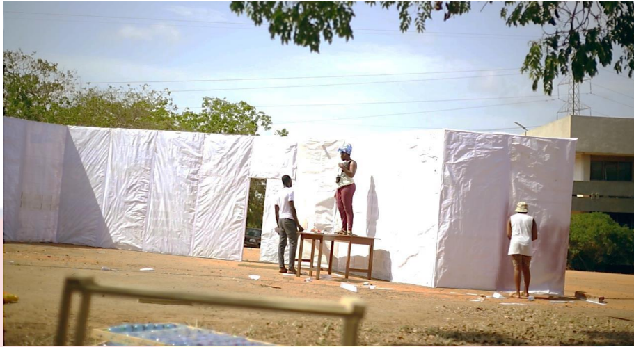
Figure 5.12. A section of the destruction caused by the gust of wind during the construction of the interior design. Picture taken by Bismark Ofori (16th April, 2021) for Mawukplorm H. Adjahoe: waste designing (2021)
