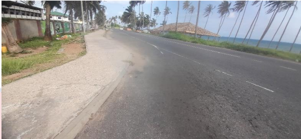
Figure 14 Concrete pedestrian lane on the Cape Coast Beach Road
