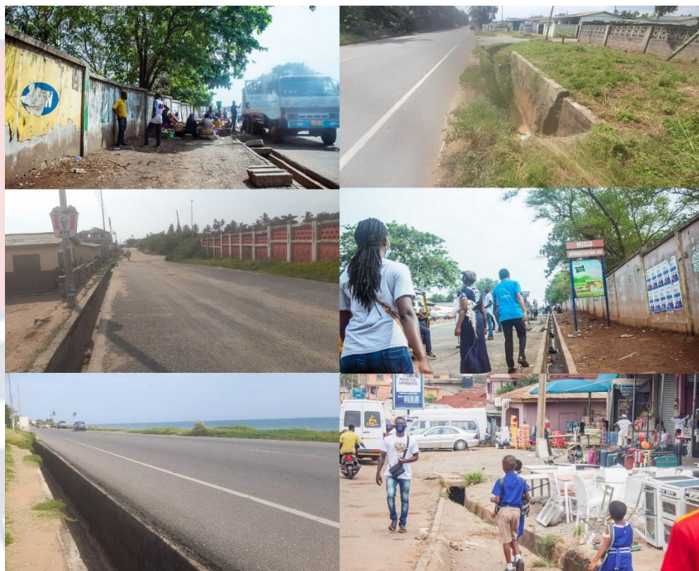
Figure 23 Images showing open drainages along routes in Kumasi and Cape Coast
