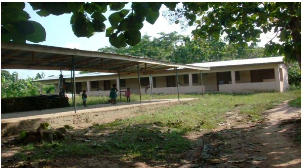
Plate 3: Health centre and nurses housing quarters under construction
