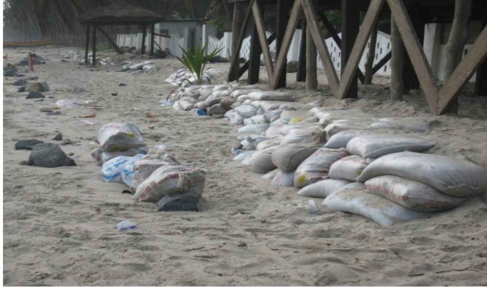
Plate 10: shows efforts being made by natives to prevent further erosion. However these efforts have been proved futile since the structures are being eroded and buried on the beach (Field Observation, 2008-2011).
