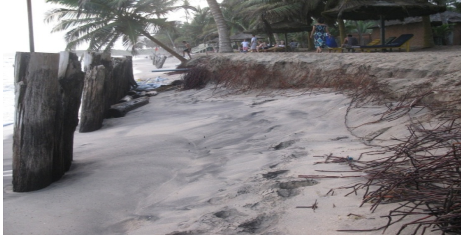
Plate 2: A picture of eroding soft cliff at Anomabo Beach Resort (Field Observation, 2008-2011). Some facilities such as summer huts and other structures are washed away as erosion continues on the beach.
