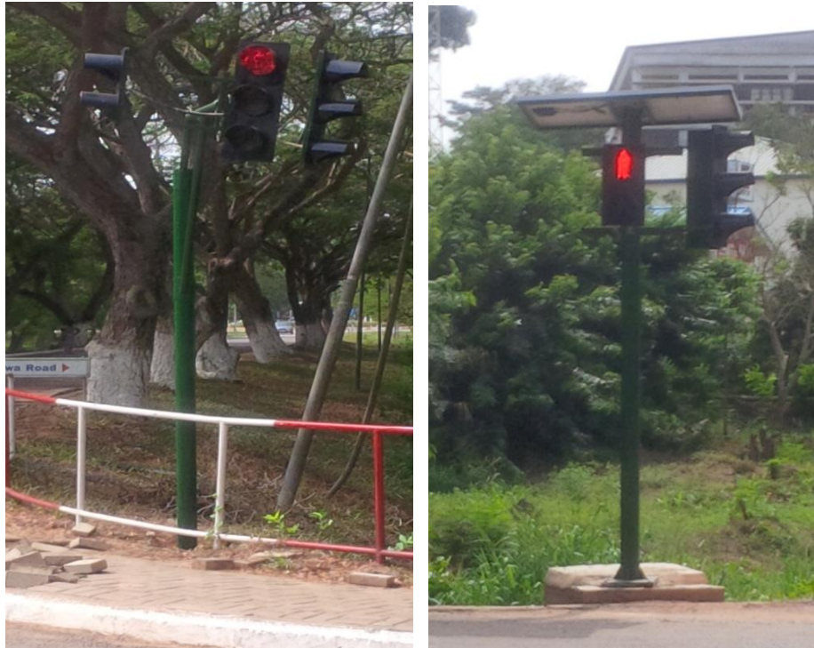
Figure 18: Traffic lights without push bells and audio transmitters close to the 4-way junction adjacent Zenith Bank.
