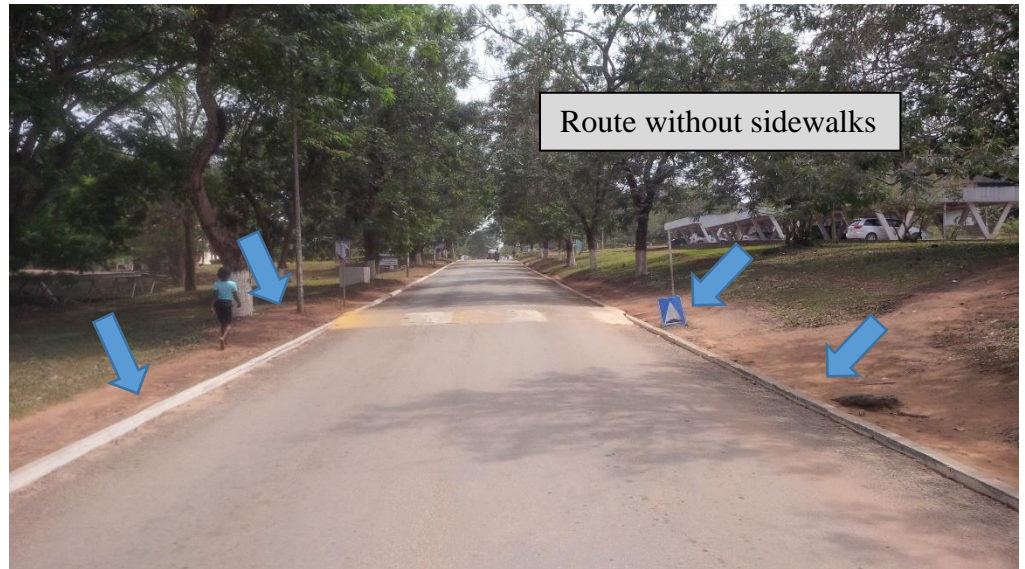
Figure 22: Route without sidewalks.
