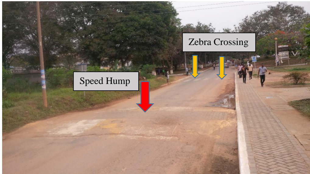
Figure 16: Speed bump before the crossing point, towards SRC hostel
