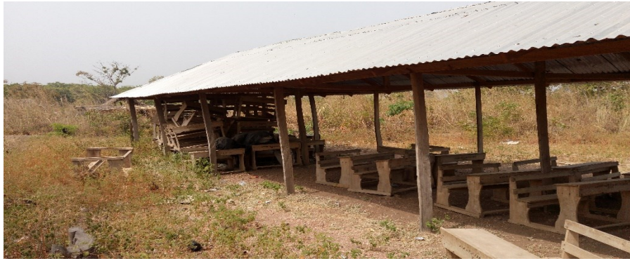
Plate 5: School Structure at Adjoining Photo Credit: Author (2017)
