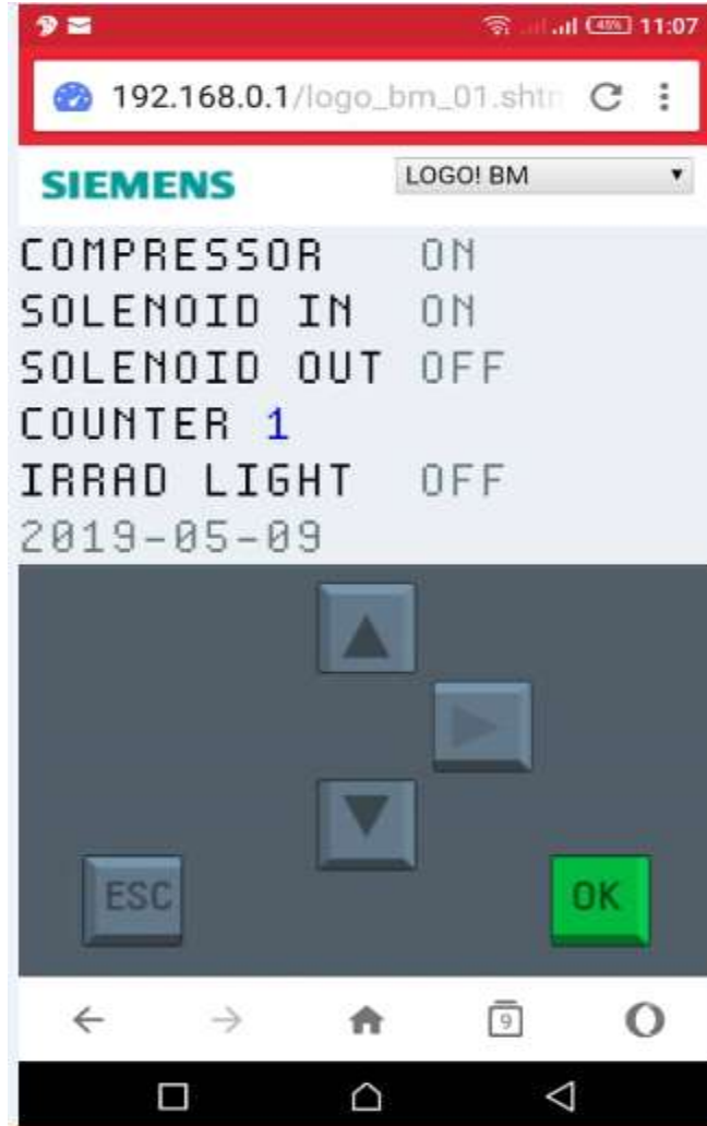
Figure 86: Air-compressor and solenoid-IN buttons depressed, compressor ON and solenoid-IN opened (monitored from mobile phone).
