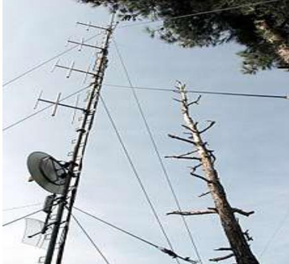
*Figure 7: A photograph of a collinear antenna array*
