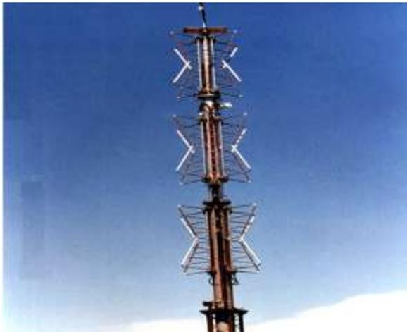
*Figure 13: A photograph of a Batwing antenna*
