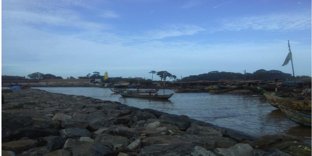
Plate 10: Construction of Sea Defense at New-Takoradi
