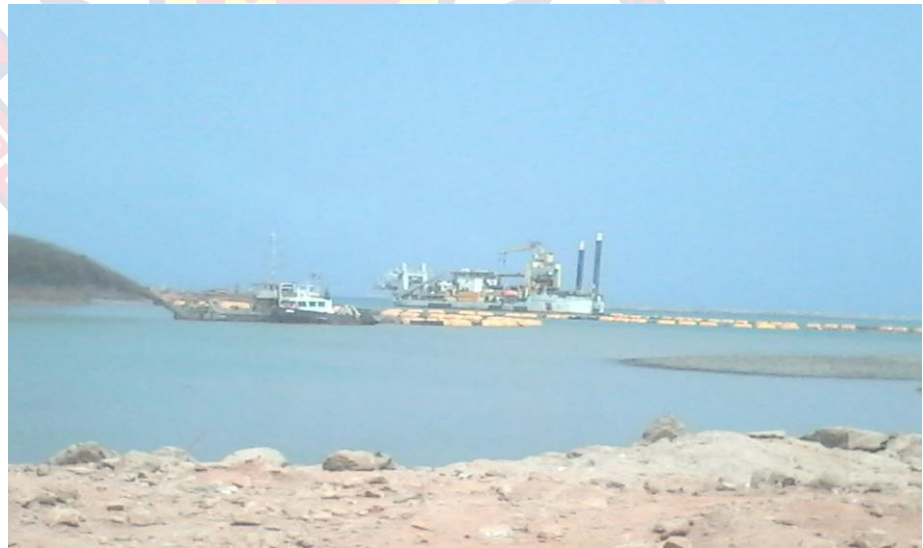
Plate 6: Takoradi Port Expansion; Land Reclamation from the Sea
