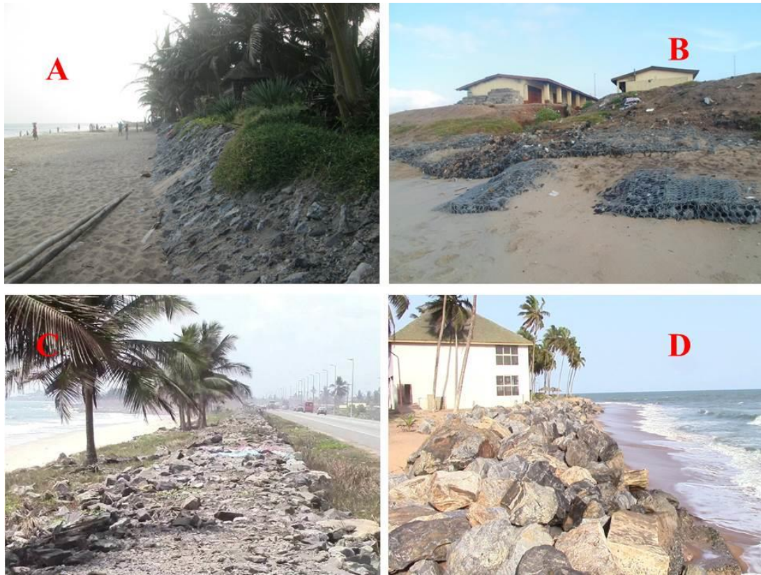
408 Figure 12: Some coastal defence structures in the study area. (A) Seawall to protect a beach 409 resort in Cape Coast, (B) wire mesh revetment to control erosion near a school facility in 410 Cape Coast, (C) section of a 1.5 km major sea defence project to protect a section of the Cape 411 Coast-Takoradi highway, (D) boulder revetment used to prevent further destruction to a 412 beach resort at a rapidly receding beach in Elmina.
